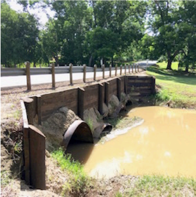
Old Culvert System
